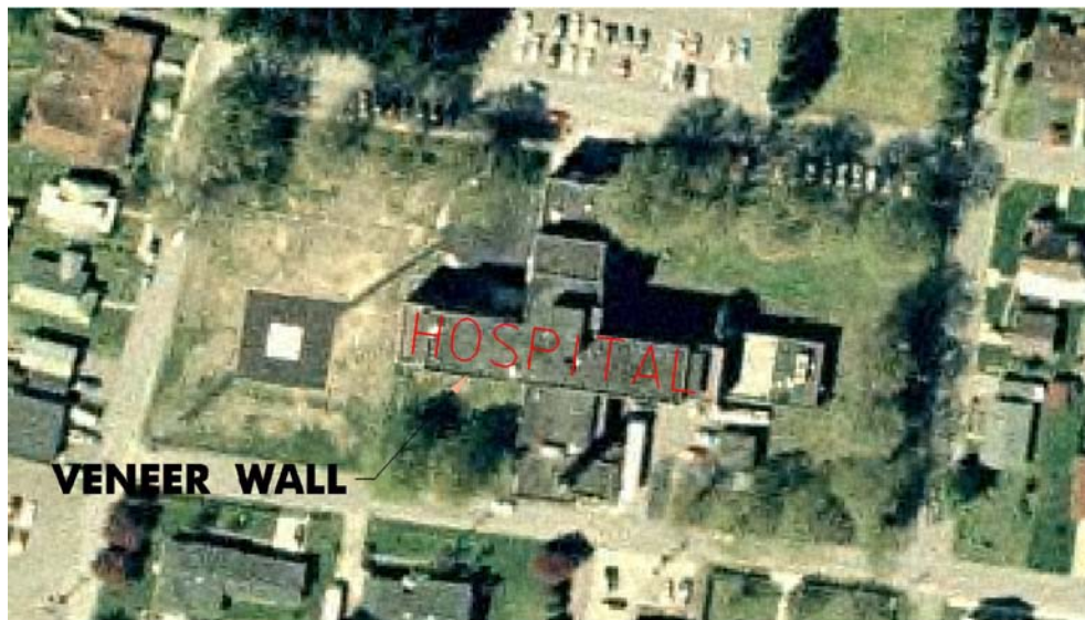
Figure 18. Hospital Veneer Wall
