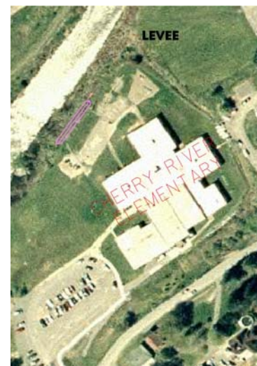
Figure 15. Elementary School Levee
